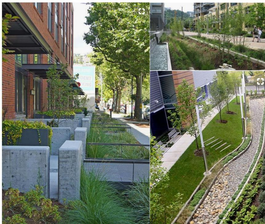
**Figure 5.1** Examples of Urban Swales/Bio-swales – Various Sources
